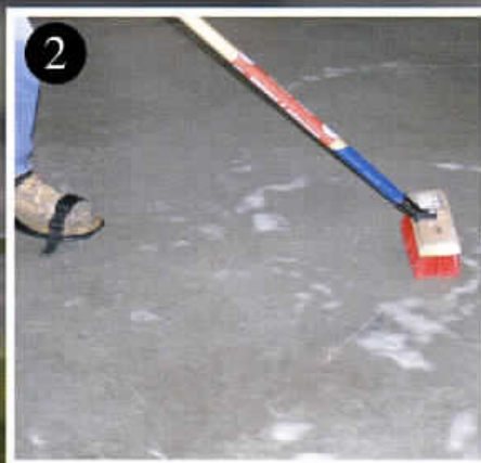
2 Scrub floor with degreaser
