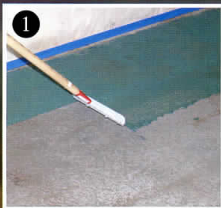
1 Scraping softened epoxy floor paint
